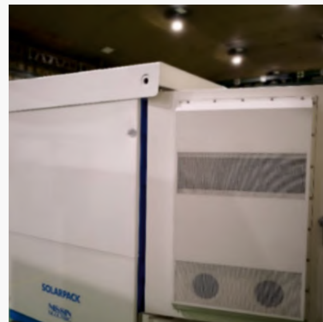
Nissin Energy Inverter Cabinet Cooling
