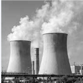
Thermal Power Plants
